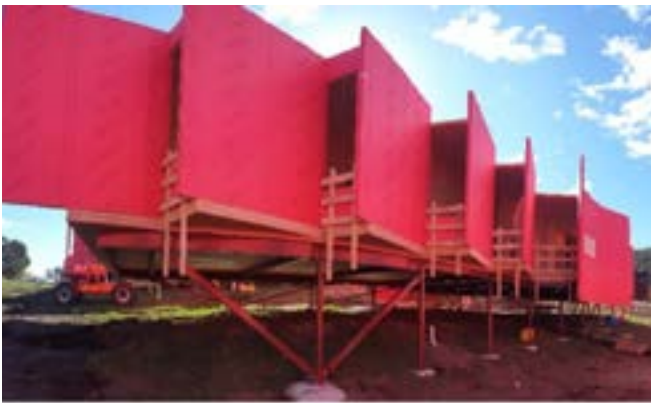
Figure 3 XLam CLT with Pre Applied Membrane
